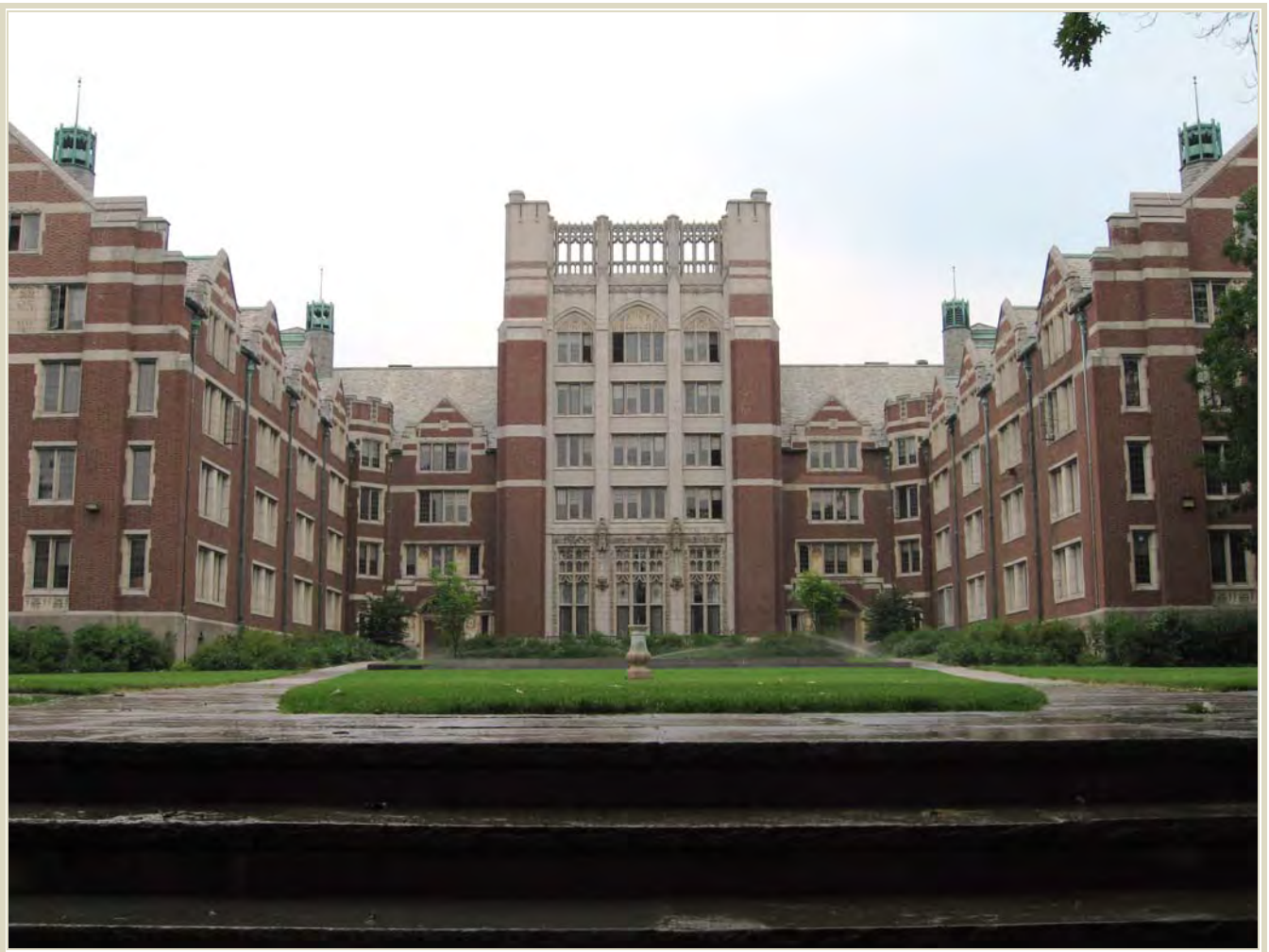
Tower Court on the campus of Wellesley College
