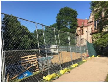
Erosion controls in place during Town Hall construction work.
