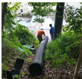
Flexible pipe is inserted into the dam upstream.
