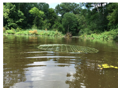
Protective cages keep beavers from getting into the pipes and
