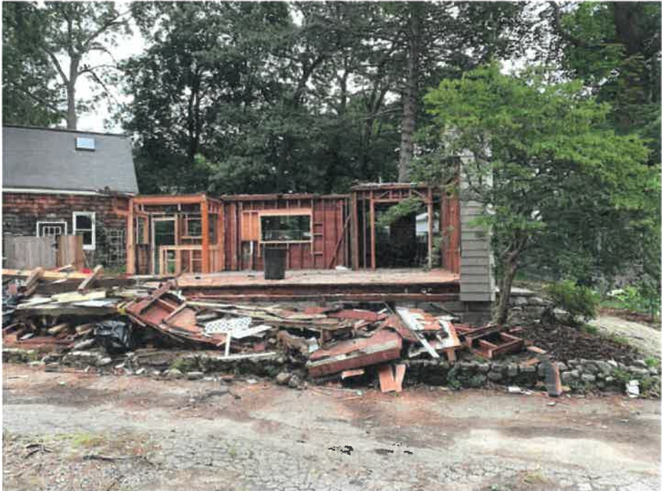
Photo of existing wall during demolition. It was not salvageable.
