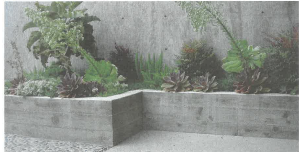
DECORATIVE CONCRETE RETAINING WALLS
