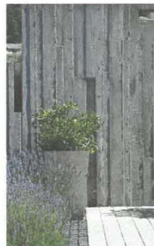
9' max Retaining Walls Vertical Board Formed Concrete Retaining Wall or Use Formliner product
