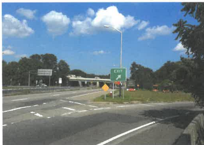
Facing view; 128 onramp
