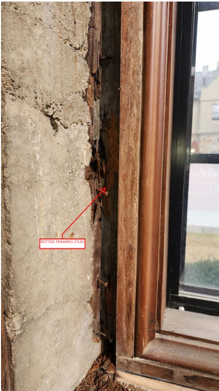
ROTTED EXISTING WINDOW FRAME
