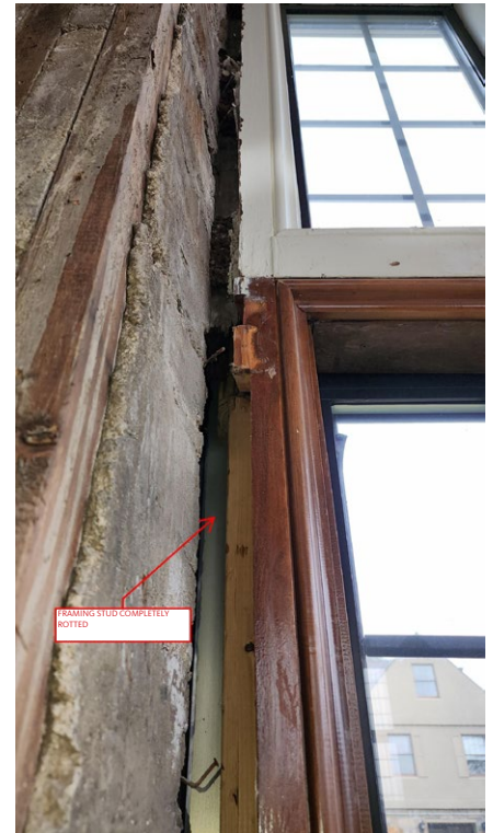
ROTTED EXISTING WINDOW FRAME
