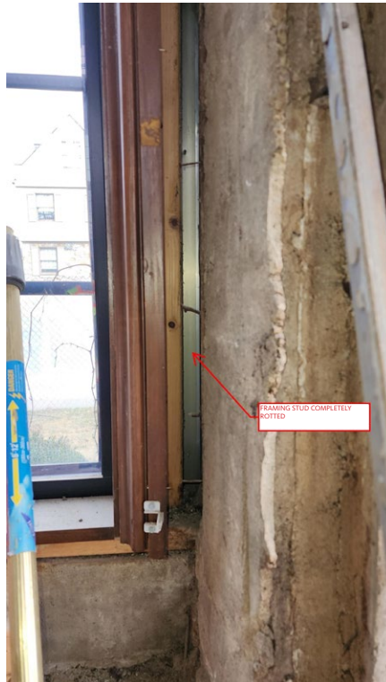
ROTTED EXISTING WINDOW FRAME
